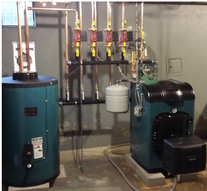
When an oil-fired boiler is used, Modern always looks to the durable, efficient, feature-rich MPO-IQ.
